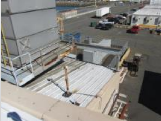
Abandoned mechanical unit
