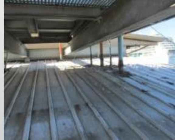
Underside of abandoned mechanical unit
